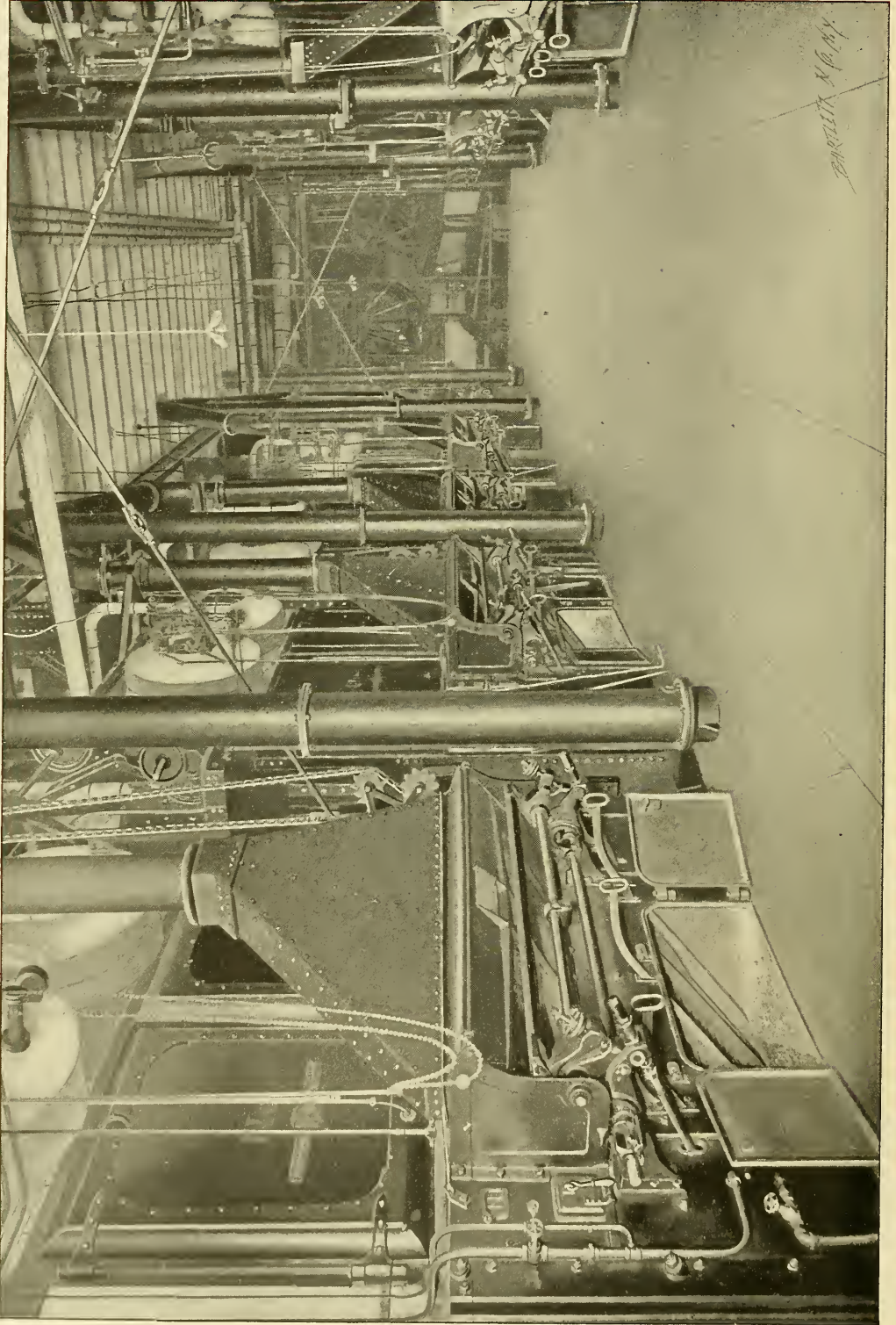
Babcock & Wilcox Boilers fitted with Roney Stokers, in 96th Street Station, Metropolitan Street Railway Co., N. Y. 60,000 H. P. in the various stations of this Company and its leased lines.
